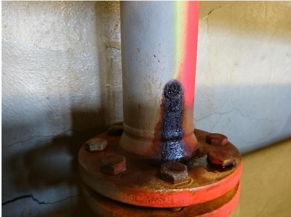
**Figure 27.** Permeate from depleted brine PTFE/steel pipeline's weep hole at the bottom of a dropdown pipe from electrolysis cell has corroded the steel substrate.
