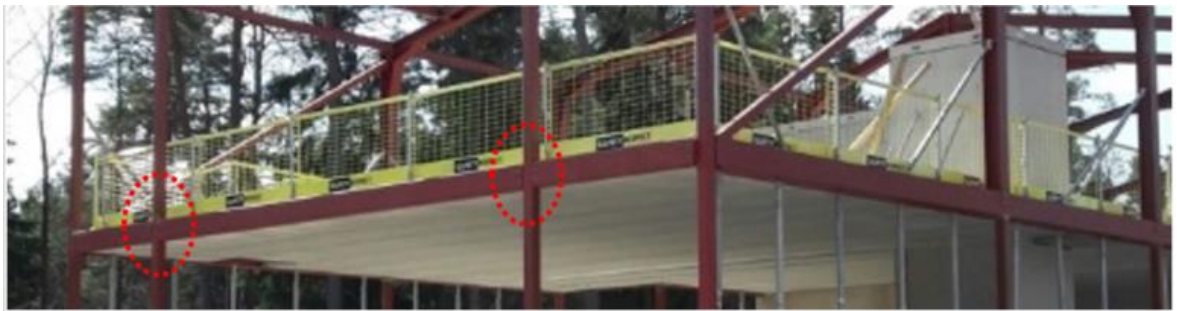
Fig. 1. Typical tubular structure with X-joints which can be subjected to axial compressive loading.
