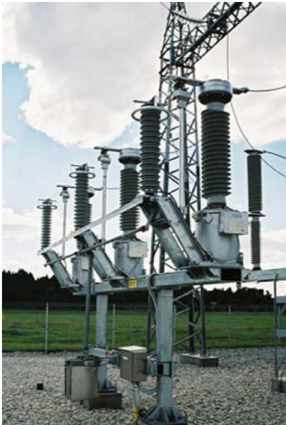
Figure 3.3 Withdrawable circuit breaker for 72.5 – 300 kV [6].
