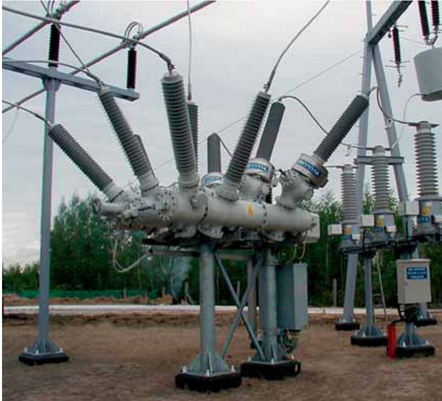
Figure 3.8 PASS M0 Double busbar. [8]
