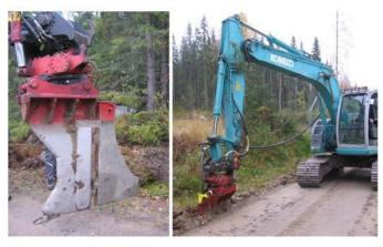
Figure 3.1. a) Cable plough b) Ploughing of AMCMK-PE -cable (Reka 2011)
