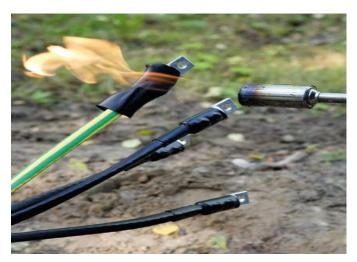
Figure 2.3. LV cable termination using lugs and heat-shrink tubes. (Ensto, 2011)
