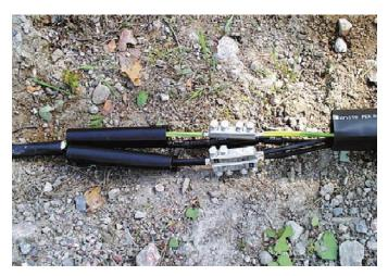
Figure 2.4. Bolted LV cable joint. Bolted connections will be protected with smaller heatshrink tubes, while larger tube serves as a sheath to whole joint area. (Ensto, 2011)
