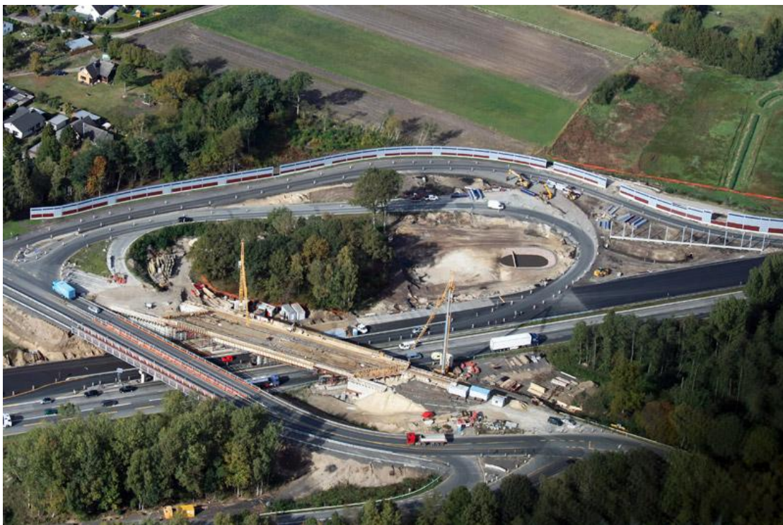
Figure 24. Aerial view of construction of BAB 1 28
