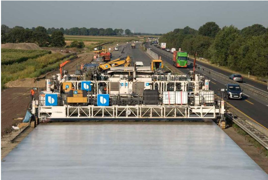
Figure 25. Construction of BAB 1 during traffic flow 29
