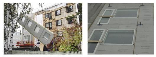
Fig. 3.1: Paroc's passive house concept is based on prefabricated facade elements with substantial insulation and energy efficient windows [Paroc, 2012b].
