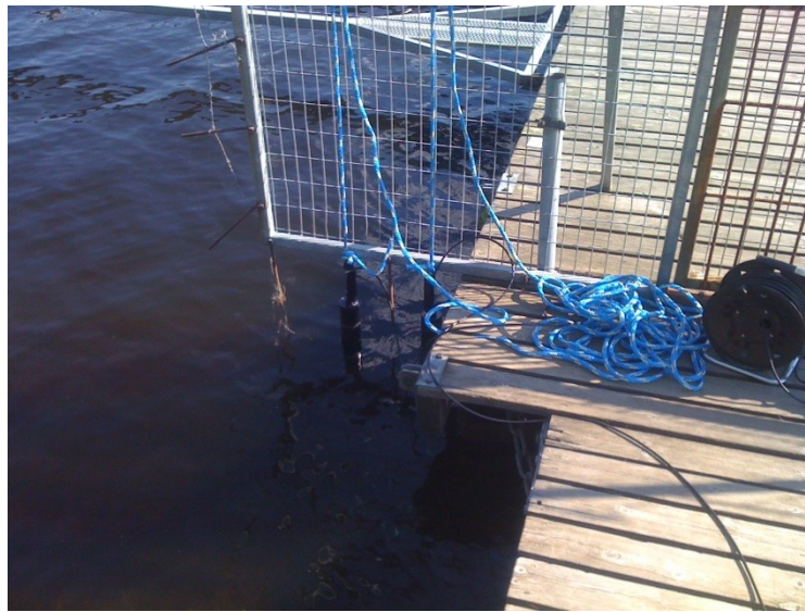
Figure 31 Installation of the probes in Tuppurala
