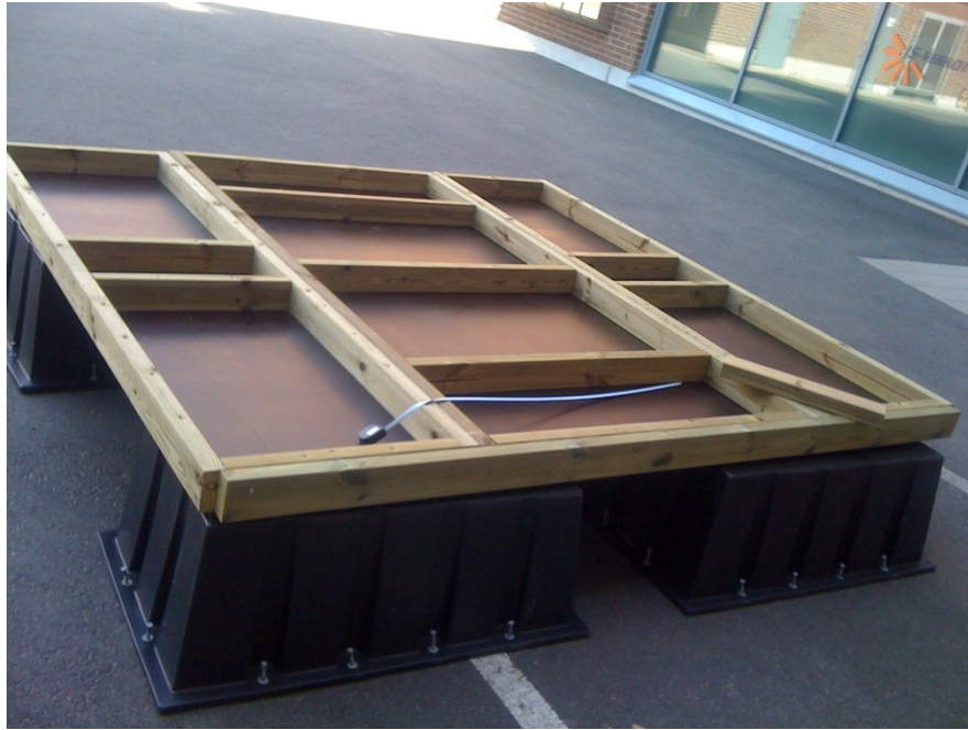
Figure 28 Construction and building up of the ferry
