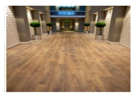
Figure 8. High Pressure laminate floor (Bisson, Deomano & Do, 2014).
