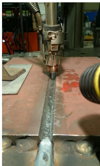
Figure 45. Angle of the welding head before welding the third bead - D35.3 with 7 degree angle between the wires and the welding direction.
