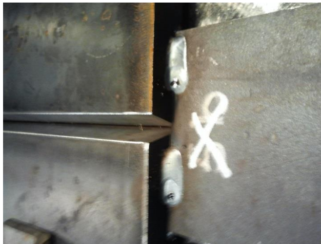
Figure 28. Work piece prior welding with 30° groove angle.
