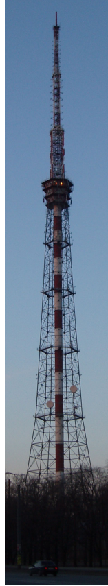
Figure 3.2: Saint Petersburg TV tower.
