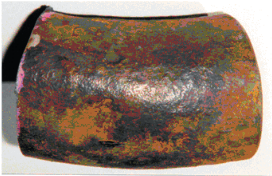
Figure 10-4, Corroded superheater tube (Suik, 2001).
