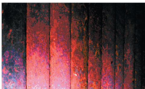
Figure 10-10, Chloride corrosion in superheater bank (Koivisto, 2000).
