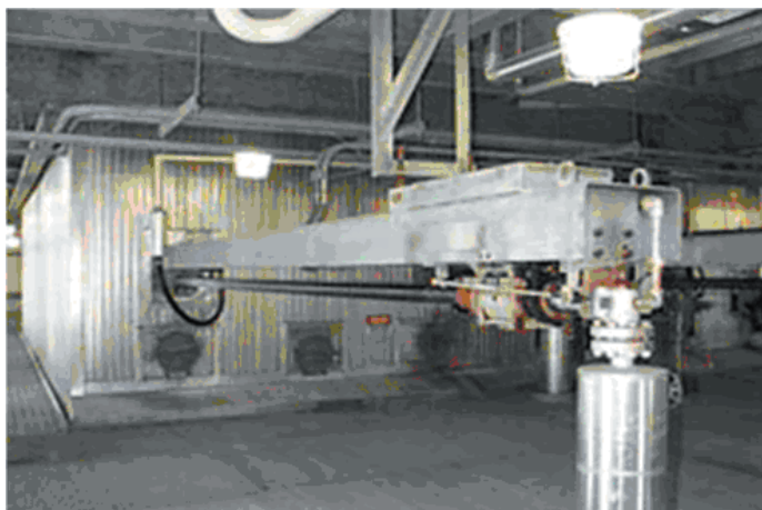
Figure 7-35, Retractable sootblower.
