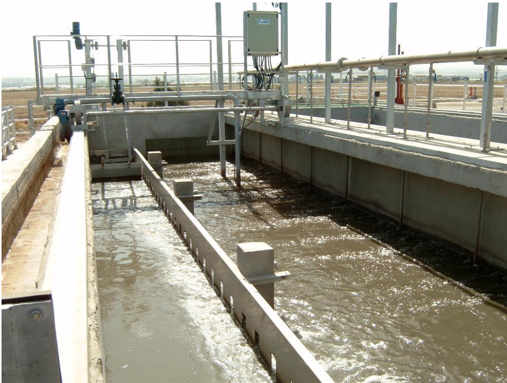
Picture 9: Grit chamber in WWTP (T.L.M Engineers 2008)
