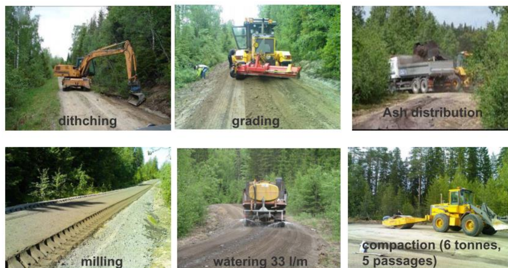
Figure 12: Upgrade of a gravel road using fly ash (Vestin, 2012).
