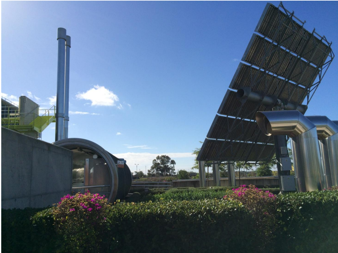
Figure 24: El Tubo installation [111].
