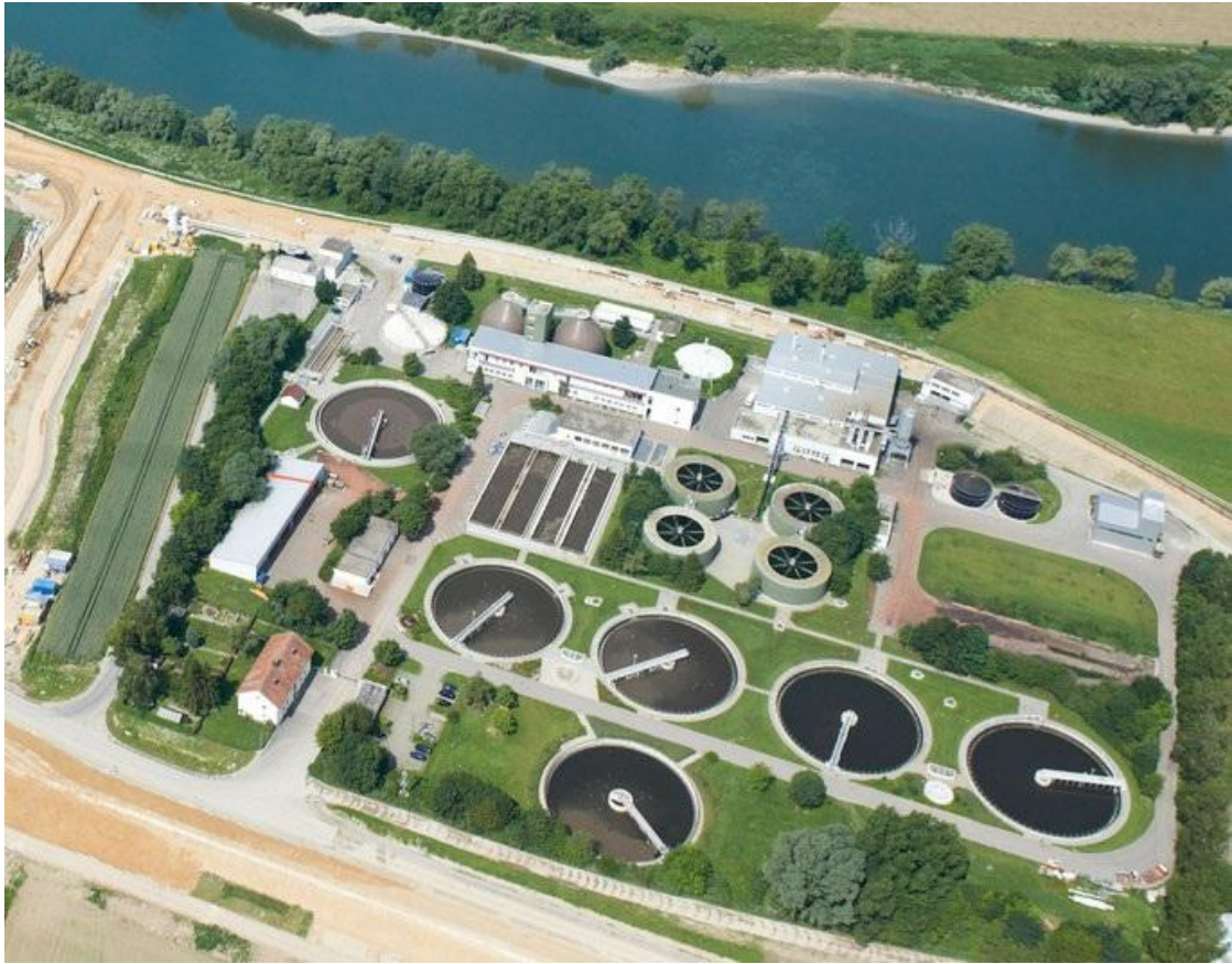
Figure 15: The water treatment facility in Straubing [71].
