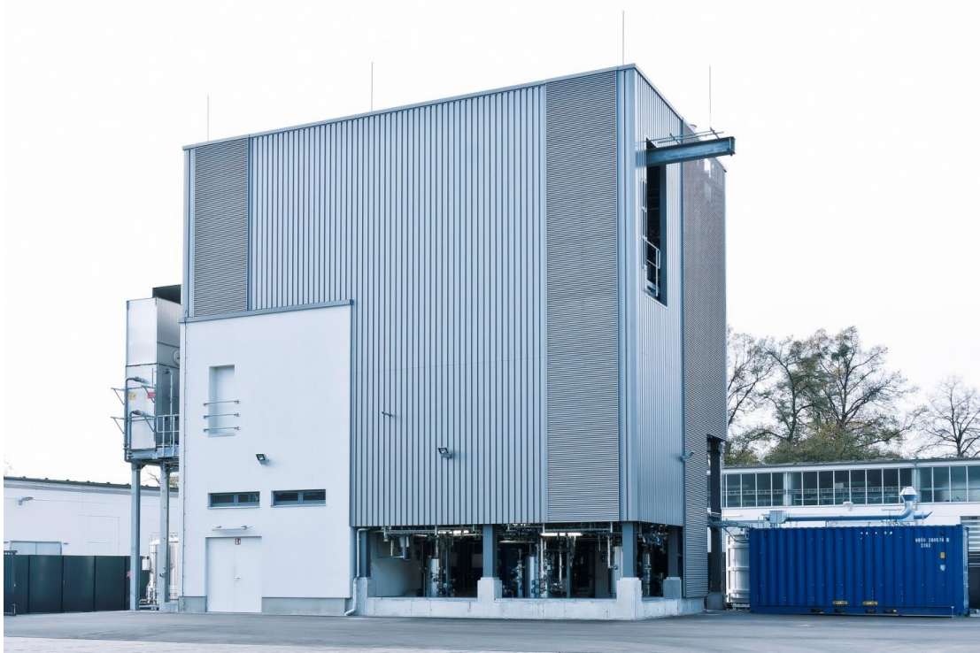
Figure 16: Power to liquid plant in Dresden [77].
