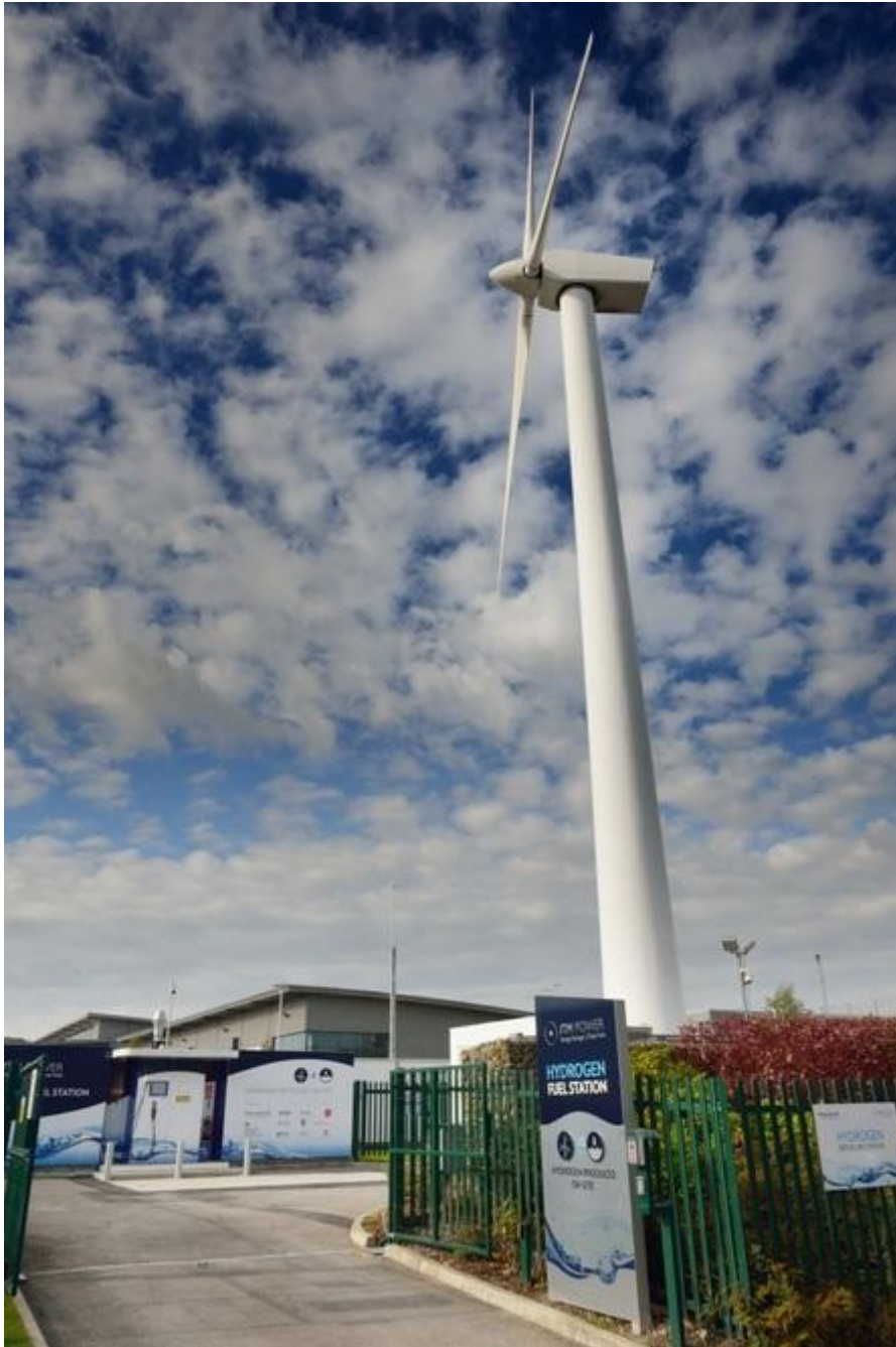
Figure 27: Hydrogen fueling station and wind turbine of the facility [131].
