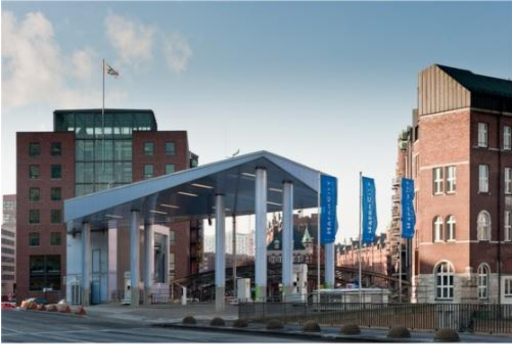
Figure 7: The Hafencity hydrogen fueling station [45].
