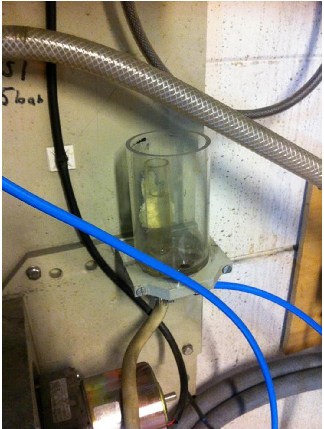
Figure 13. Sample basin is the smaller cylinder in the middle, feed is from the bottom. Container surrounding it works as a drain to remove excessive sample from the basin.
