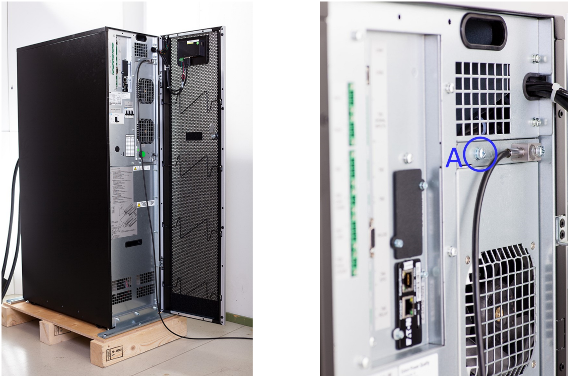
Figure 4.2: On the left the front view of UPS unit. On the right the sensor location on the front panel with a screw to be removed highlighted with blue circle. The screw is labeled A for identification.
