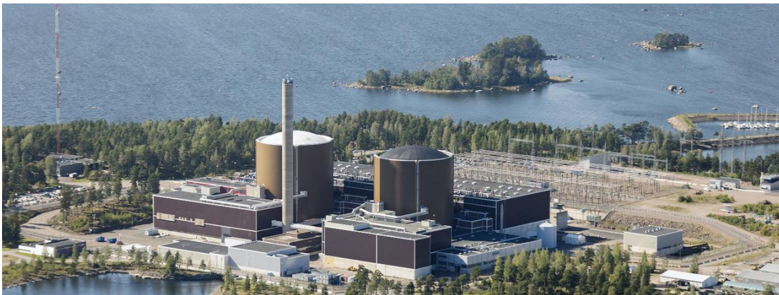
Figure 2.1. Aerial view of the Loviisa NPP (Fortum 2019)
