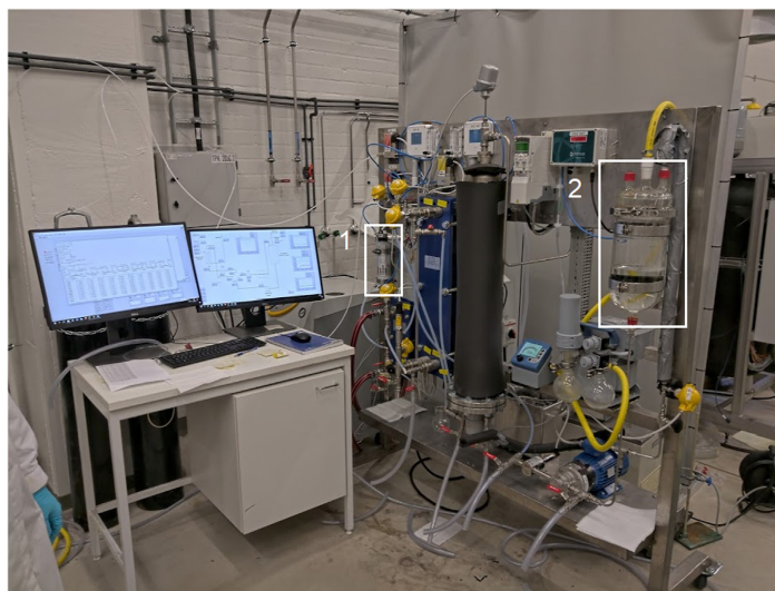
Fig. 2. Photograph of the CO 2 capture unit. 1. Membrane contactor, 2. vacuum desorption vessel.
