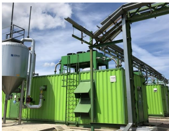
Figure 8. Landfill gas combustion units at Novyy Svet landfill (Gatchina municipality of Leningrad region, 2018)
