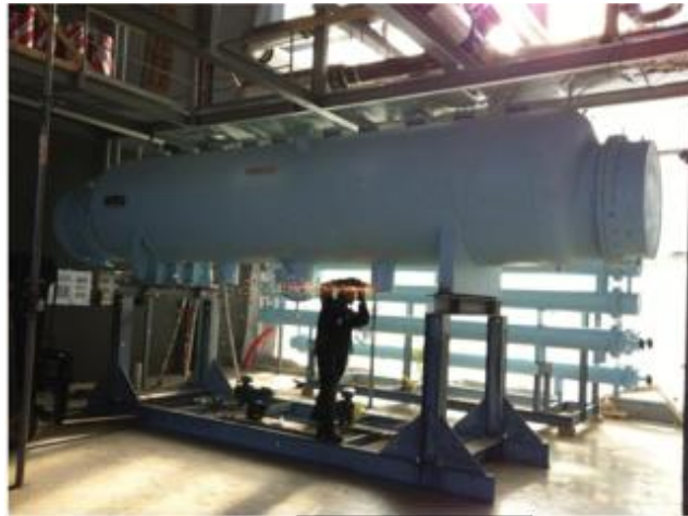
Figure 38. Spray evaporator during installation. (Zahid, 2016)
