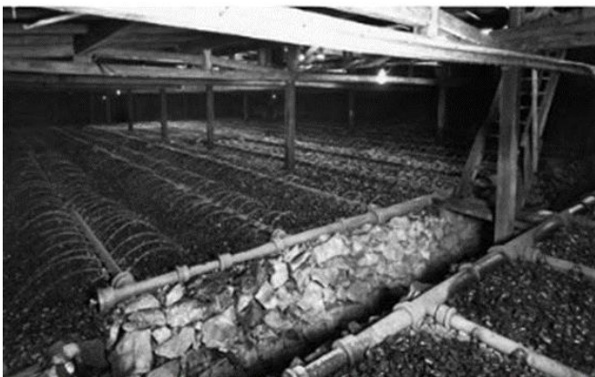
Figure 2: Alppila wwtp Gravel filter (picture Roos 1941, as cited in (Juuti, 2010))
