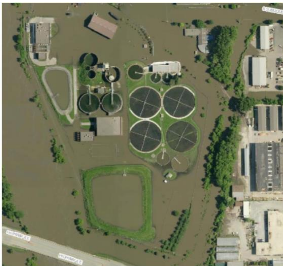
Figure 9: Flooding IA North wastewater, Iowa city WWTP after Hurricane in 2008, USA ( Iowa Homeland Security and Emergency Management, 2008).
