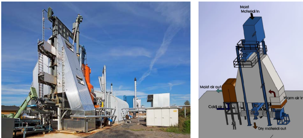
Figure 2. The pilot plant of Torrec Ltd. in Mikkeli, eastern Finland, which is a batch process where drying and torrefaction occurs inside the same reactor
