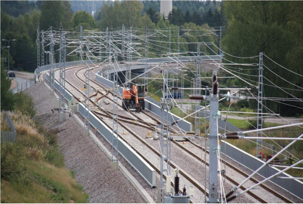
Figure 3.13: Low-height noise barrier (85 cm height) in trial use in Finland (Liikennevirasto, 2017)
