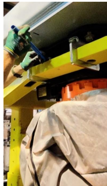
b) The robot is attached to the steel support structure.
