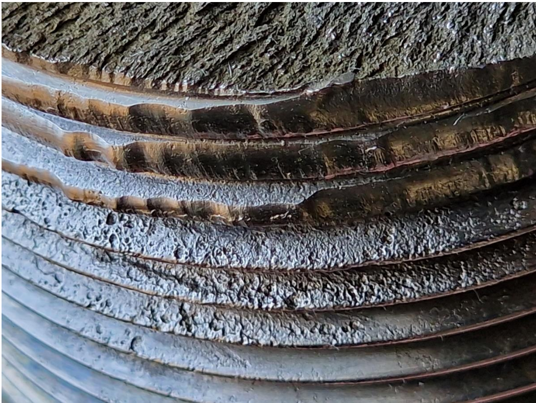
Figure 23. Corrosion in the threads of the broken bolt.
