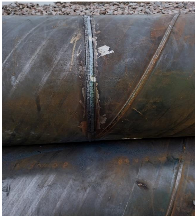
Figure 14. Continuation welding horizontally.
