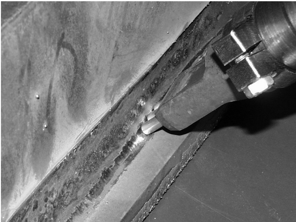
Figure 3.3 Ultrasonic impact treatment of a weld toe in progress
