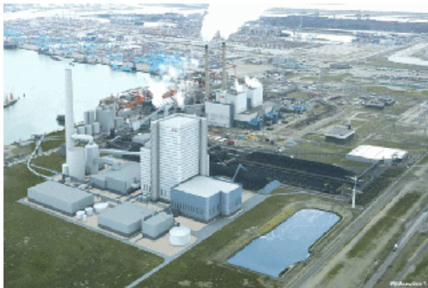
Picture 13. Co-firing of coal and MBM in E-ON power plant at Maasvlakte, Netherlands /41/.
