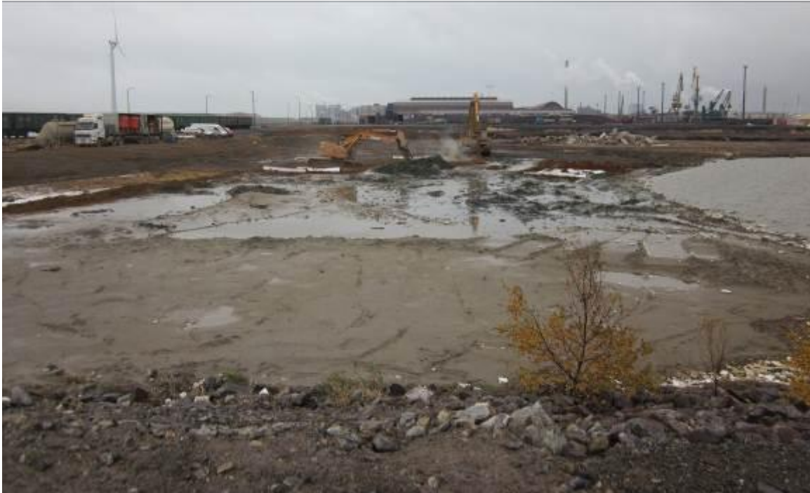
Figure 7.9. Stabilization progresses in the pool October 6, 2011.
