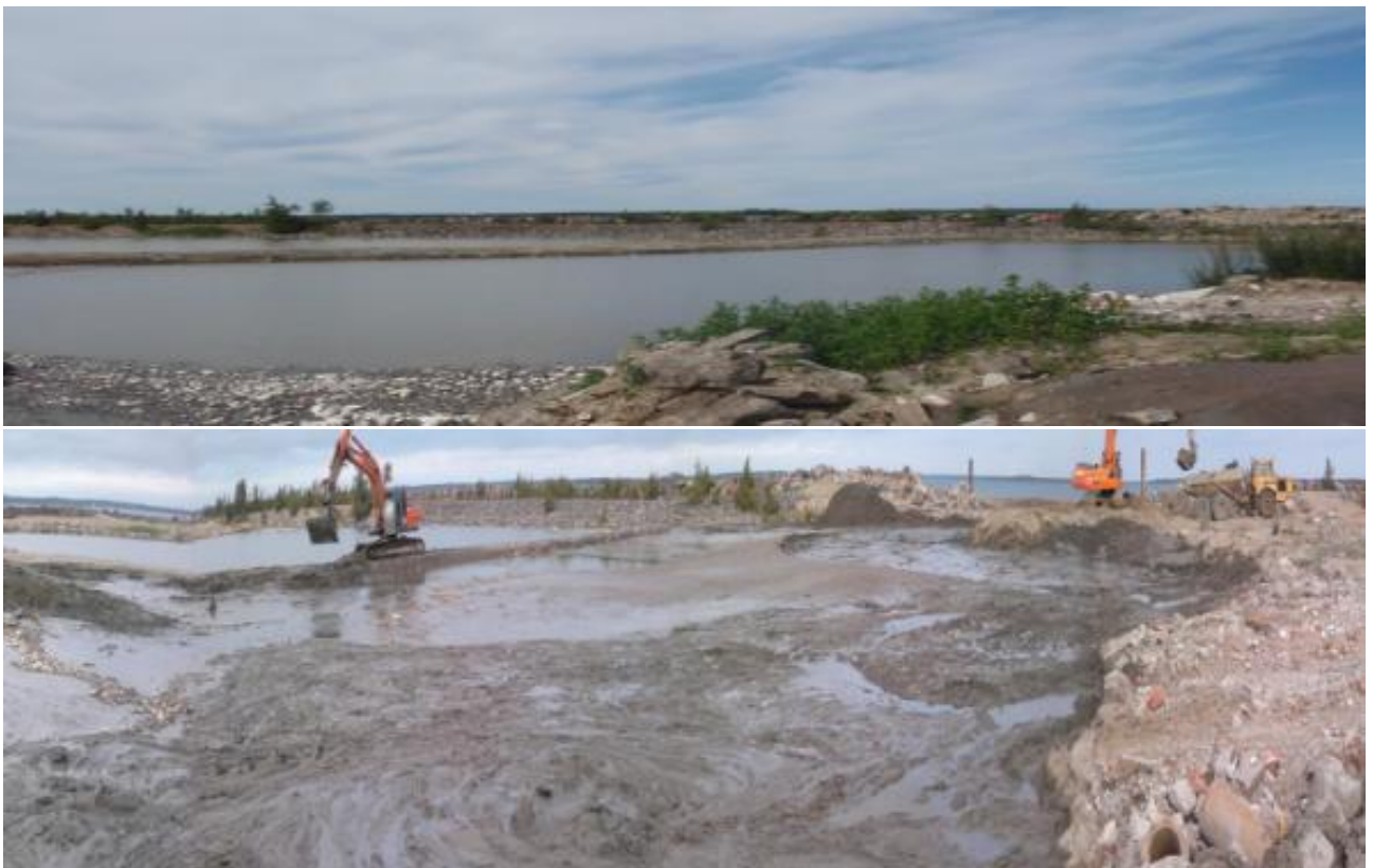
Figure 7.5. Dumping basin before and after the dredging and dumping works.
