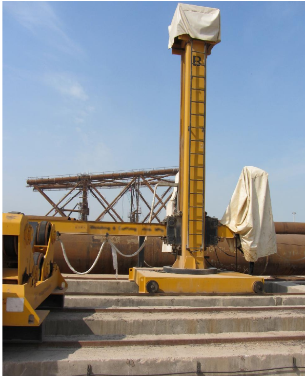
Figure 2 Column and boom manipulator use with SAW process [23]
