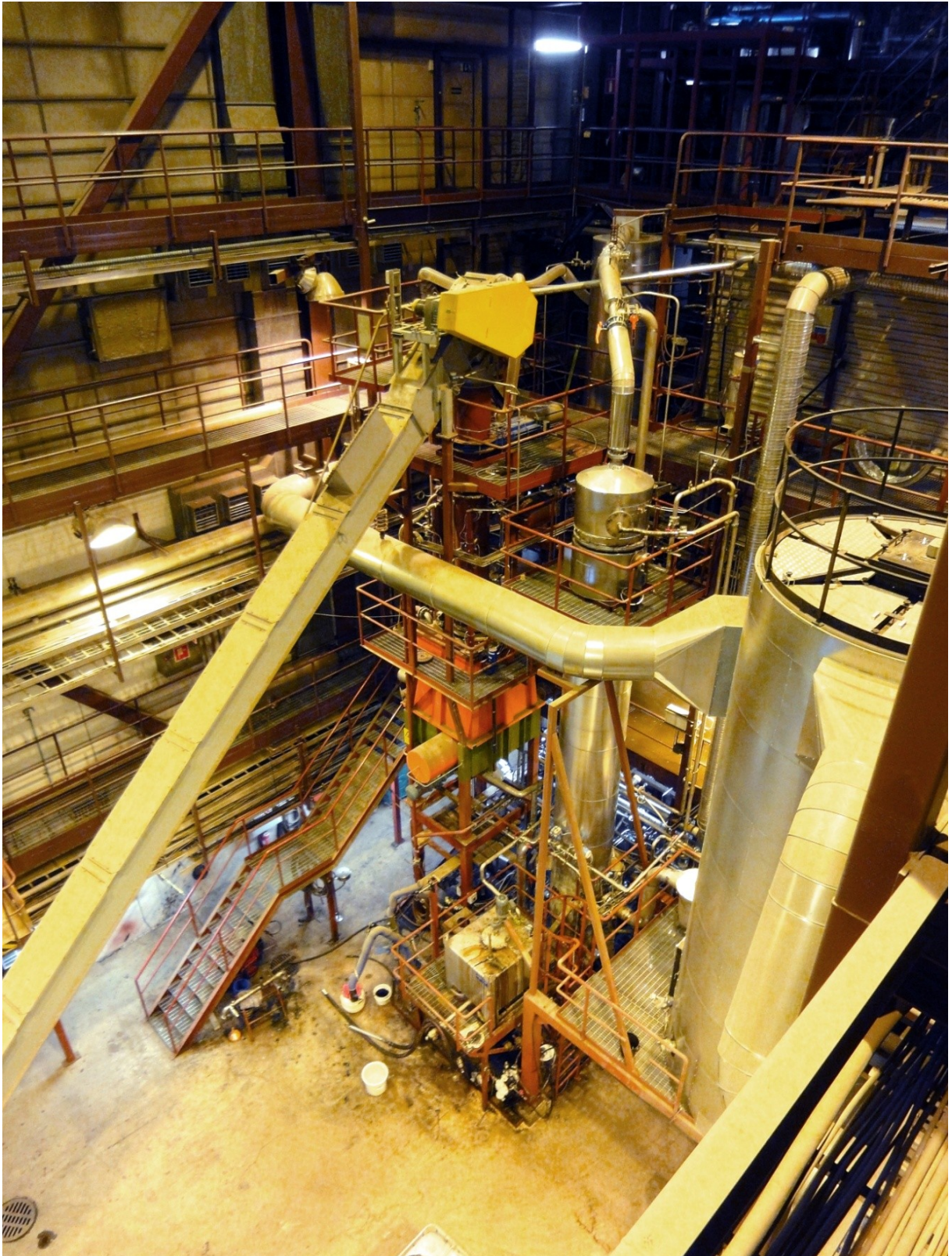
Figure 17. Part of the pyrolysis pilot plant. The fuel feeder is on the foreground, leading to the lockhopper. On the right side of the lockhopper, the gas duct from the scrubber to the condenser is seen and below it is the condenser. Next to the condenser, the product oil container is seen. The large vessel on the right is the bag house filter of the boiler.
