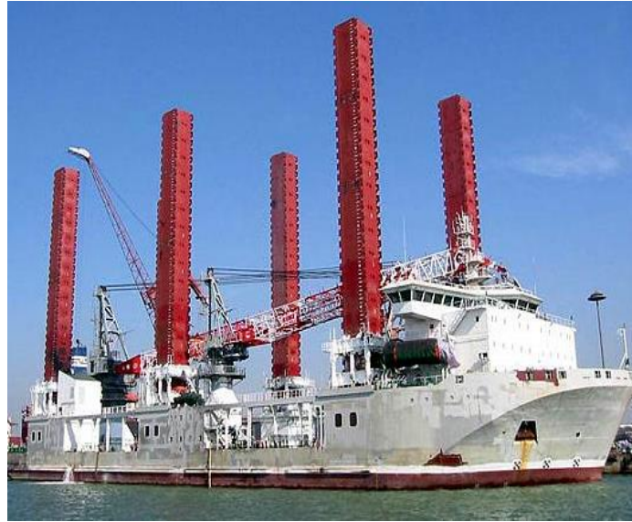
Figure 10 The Mayflower TIV- Offshore windmill constructed [41].
