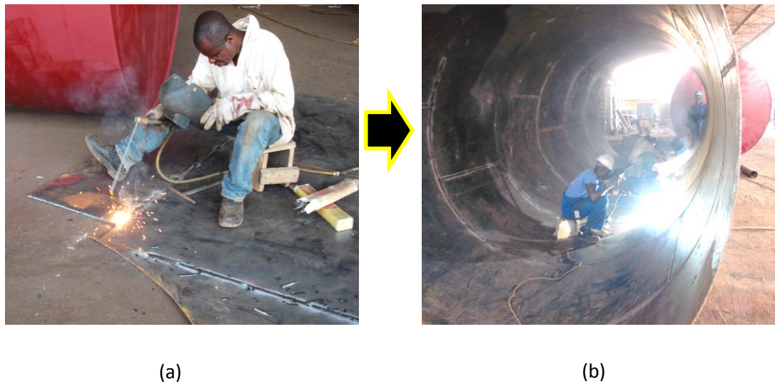
Figure 13. Welding operation utilizing manual welding technique.
