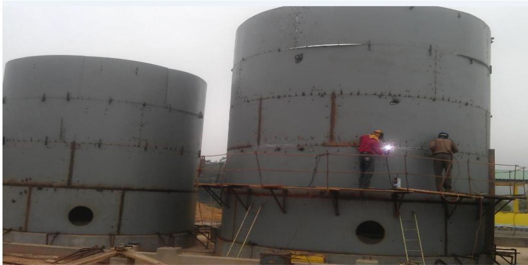
Figure 19. Water tanks construction on- site by Enas Engineering.
