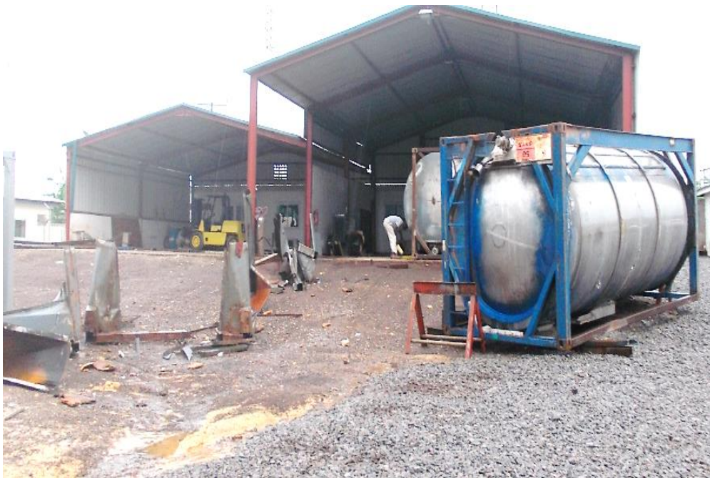
Figure 27. Swaako Engineering welding workshop.
