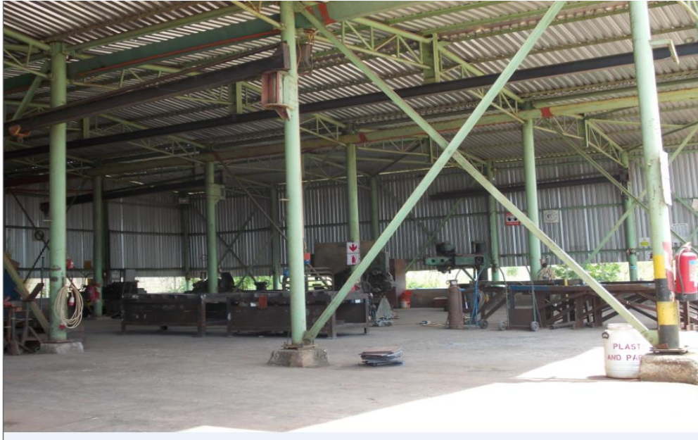
Figure 20. Group Five welding workshop.
