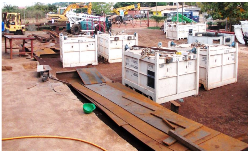
Figure 30. Wayoe Engineering material handling and storage facility.
