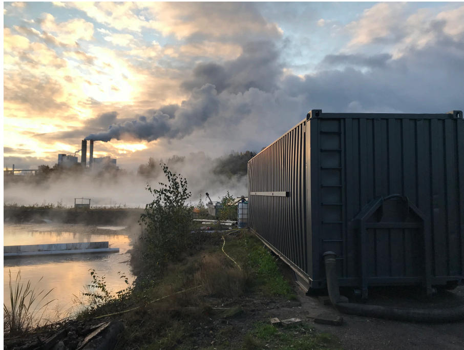
Figure 32. 55 m 3 container for reject water in mill 1 (reject water flows through the yellow tube to WWTP).
