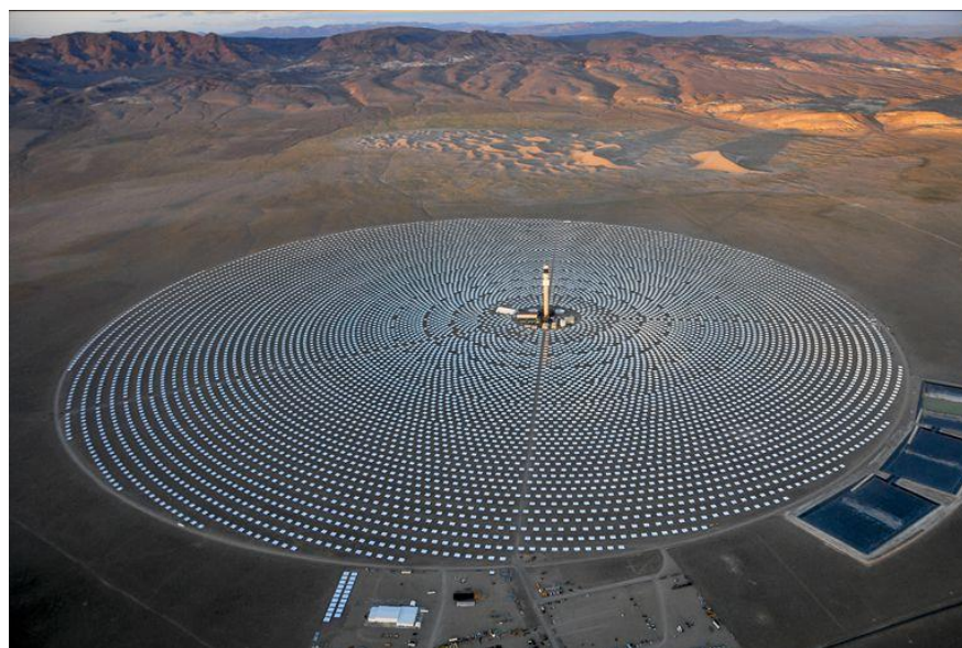
Figure 2.14: The Crescent Dunes solar thermal power plant (Solar Reserve)
