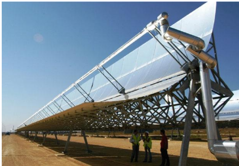
Figure 1.2: Parabolic trough collector (Richter et al., 2013, 134)
