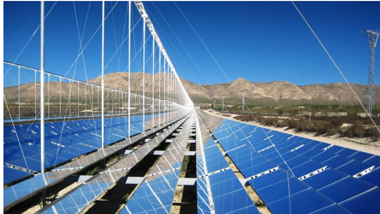
Figure 1.3: Linear Fresnel reflector (Altanova-Energy).
