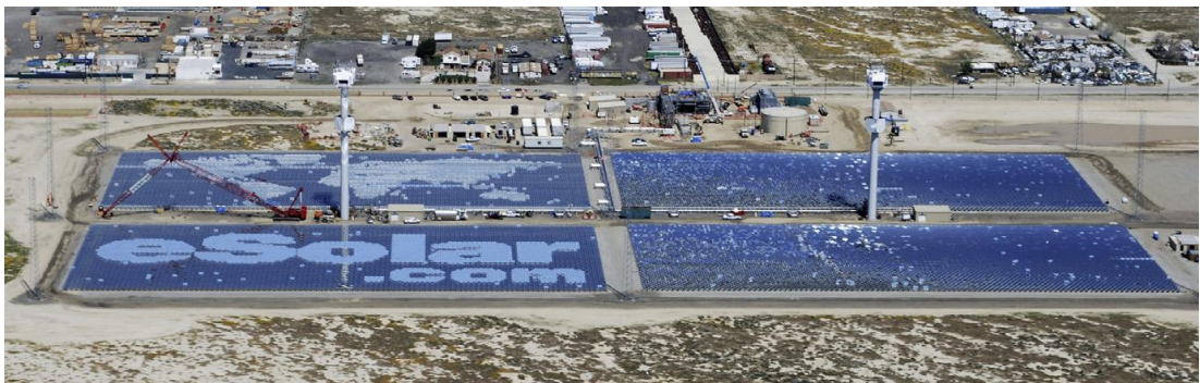
Figure 2.15: Sierra Suntower demonstration facility, Lancaster, CA, USA. (Schell, 2011,615)
