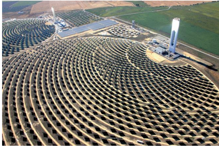
Figure 2.13: Planta Solar power plants PS10 and PS20 with north field (Müller-Steinhagen,2013,13)
