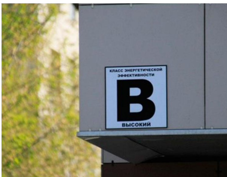
Figure 23. Indication of the energy efficiency class on the façade of apartment building ( www.dom43.ru ).
