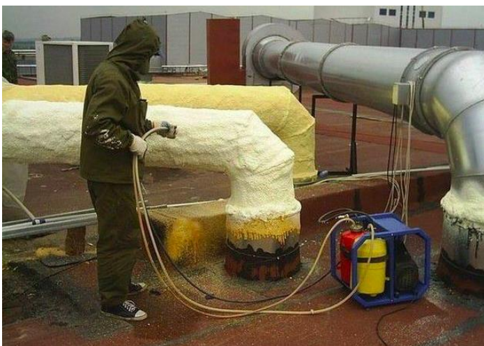
Figure 22. Spraying polyurethane foam with use of special equipment ( www.stroyday.ru ).
