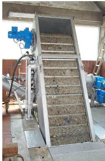
Figure 14 Example of a step screen used in municipal solid removal. (Huber Technology)
