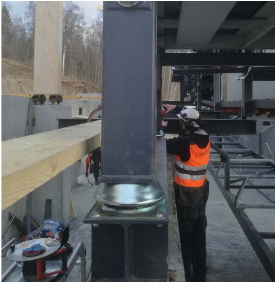
Figure 26. Vibration pad installation.
