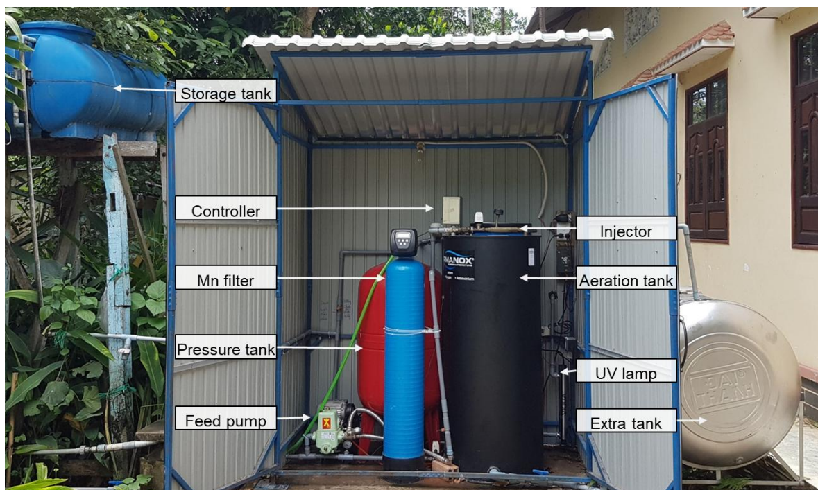
Figure 1: SAR pilot plant ( FERMANOX®-Wasseraufbereitung type BV 45 ) in An Giang, Vietnam, incl. delivery pump, pressure tank, Mn-filter and UV-lamp for post-treatment
