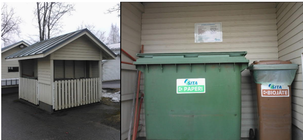
Figure 6. A waste collection shelter for recyclables and residual waste on the yard of a row house in Finland. Paper and organic waste (biowaste) collection bins in one side of the shelter. Two shelters include bins for residual waste, paper, plastic packages, biowaste, cardboard, metal and glass.
