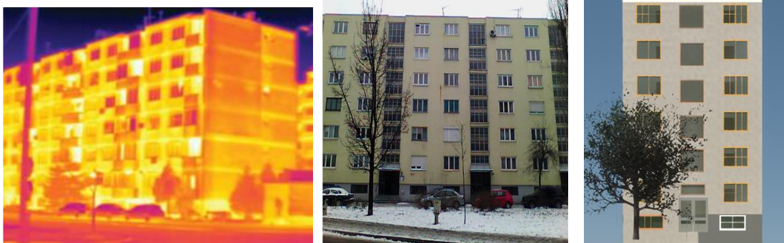
Figure 5.2. Selected residential building (from left to right: thermal image, photo, Revit 5 model)
