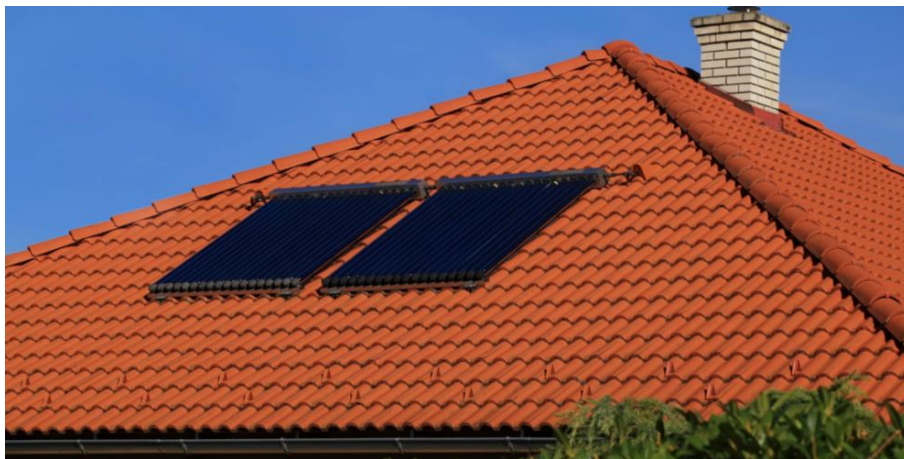
Figure 13. Solar panels on private residence adopted from [42].
