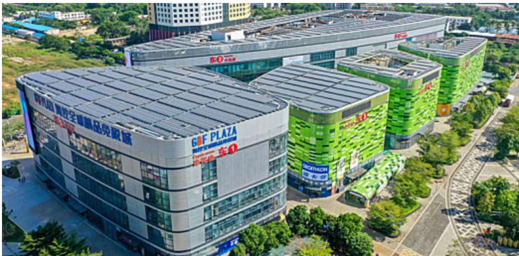
Figure 14. Solar panels installed on commercial buildings adopted from [44].
