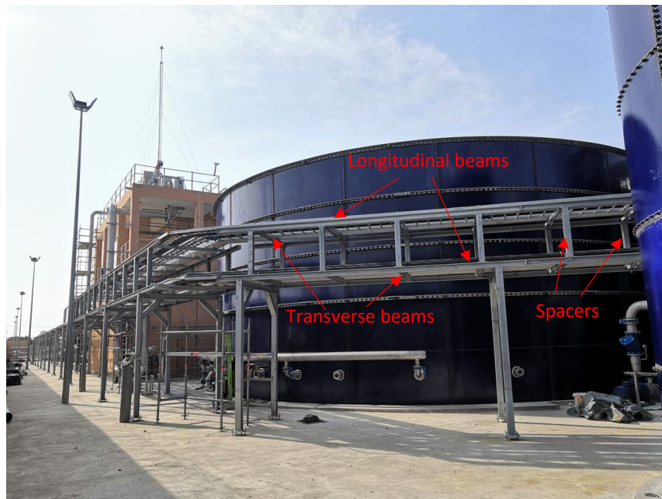
Figure 2. Pipe rack details (Stijn Vanderhulst).
