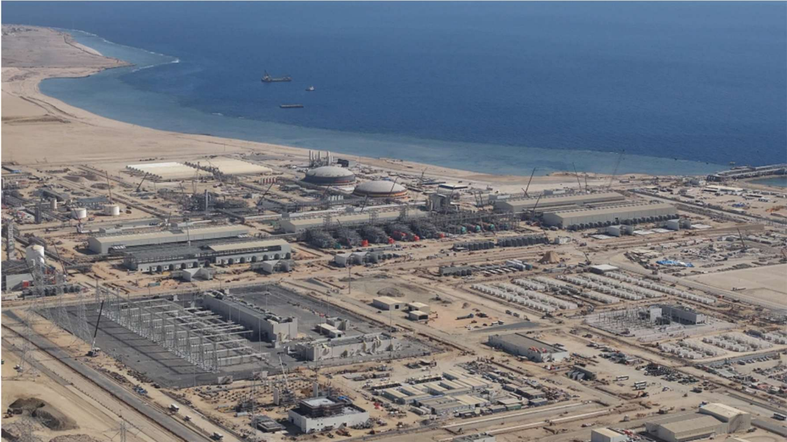
Figure 1. NEOM Green Hydrogen plant (NGHC, 2025).
