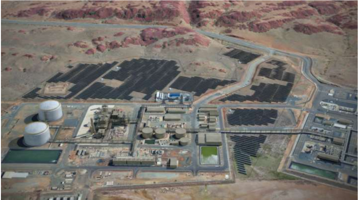
Figure 3. Yuri ammonia production facility in Karratha (ENGIE, 2022).
