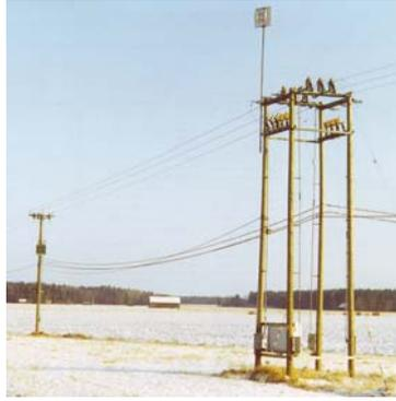
Figure 4. Remote-controlled disconnector.
