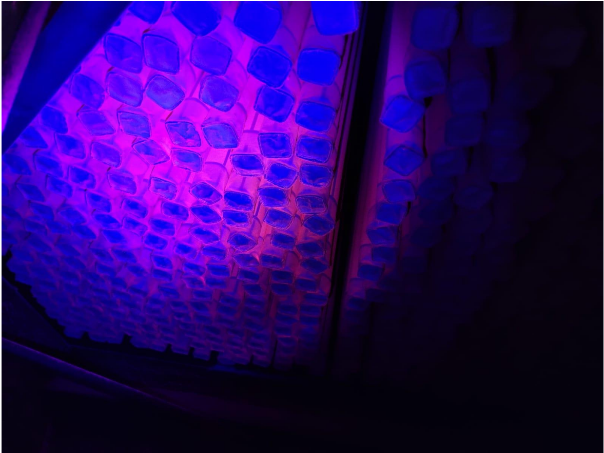
Figure 14. Bag filter leak testing on the dirty side with fluorescent powder (Valtteri Liimatainen).
